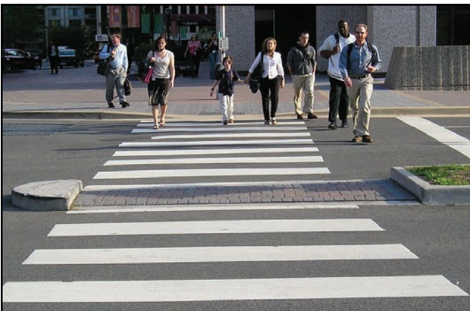
A median nose reduces the exposure time experienced by a pedestrian in the intersection
