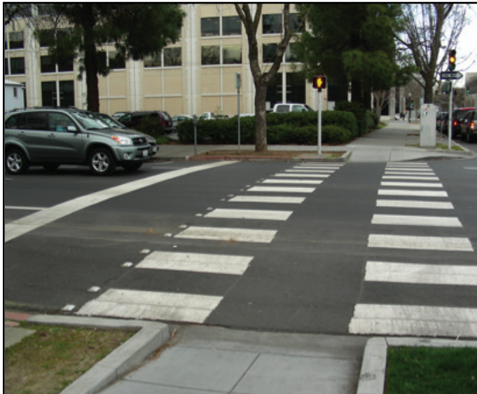
Car stops at advanced stop line, prior to crosswalk
