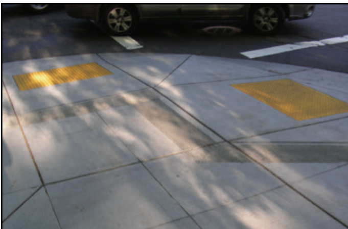
Perpendicular ramps with truncated domes assist sight-impaired and wheelchair users
