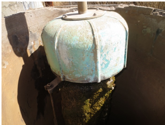
Inside Feature 3: Water Pressure Regulator (top and bottom)
