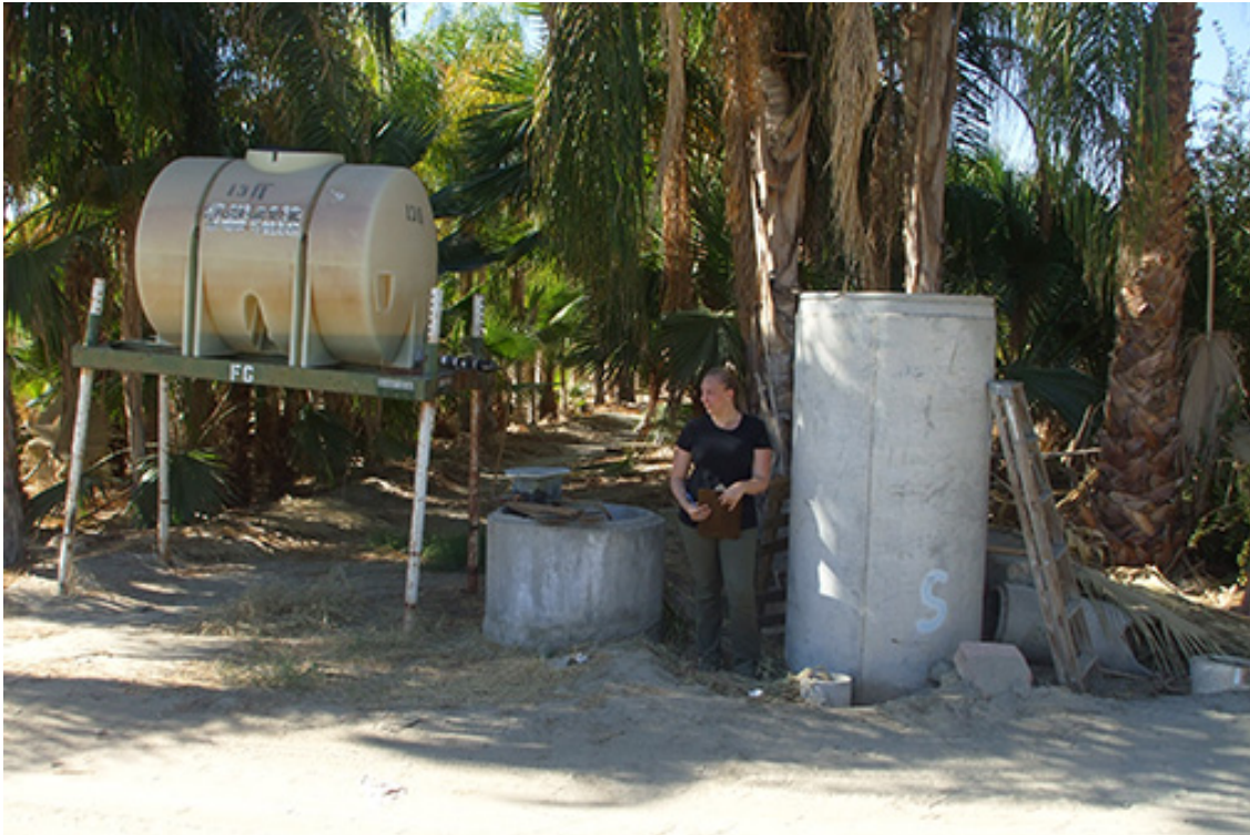
Locus F Overview facing Southwest, left to right : water storage tank (#5), well (#4), water pressure regulator with adjacent pressure relief valve (#1 & #3); and water flow gauge (#2)
