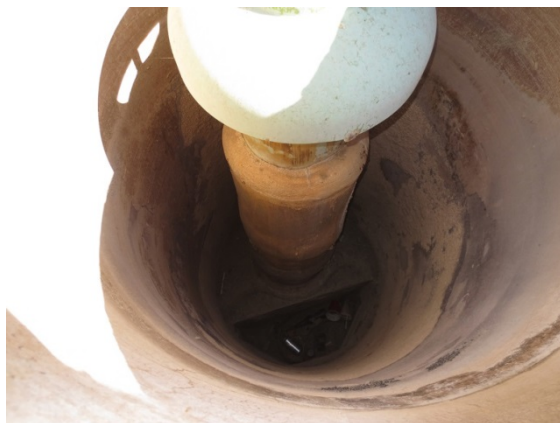
Two Views Inside of Feature 3: Water Pressure Regulator
