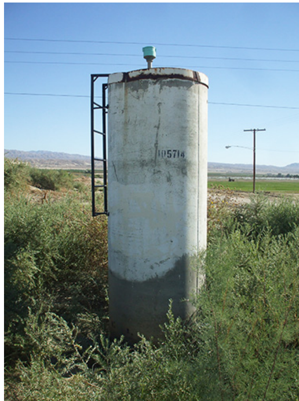
Photo 32: Locus B of RIV-11817 – Standpipe with Ladder and Water Pressure Regulator, facing roughly to the southeast
