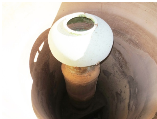
Two Views Inside of Feature 3: Water Pressure Regulator
