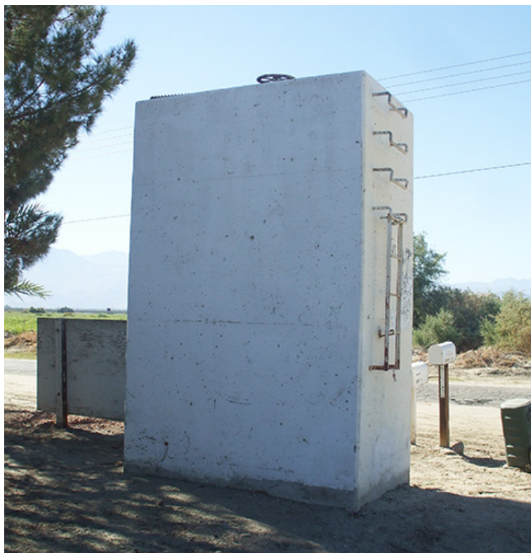
Standpipe showing Ladder and Large Valve Handle at Top, Facing SW
