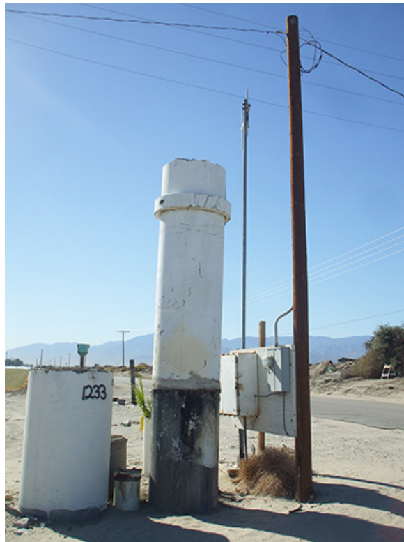
Locus A facing SSW (left to right): #3 (water pressure regulator); #2 & #4 (water flow gauge with abandoned feature in background); #1 (standpipe); and #5 (electrical panel with kW meter)
