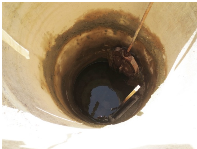
Feature 5: Probable Valve Box showing part of Valve and Valve Handle
