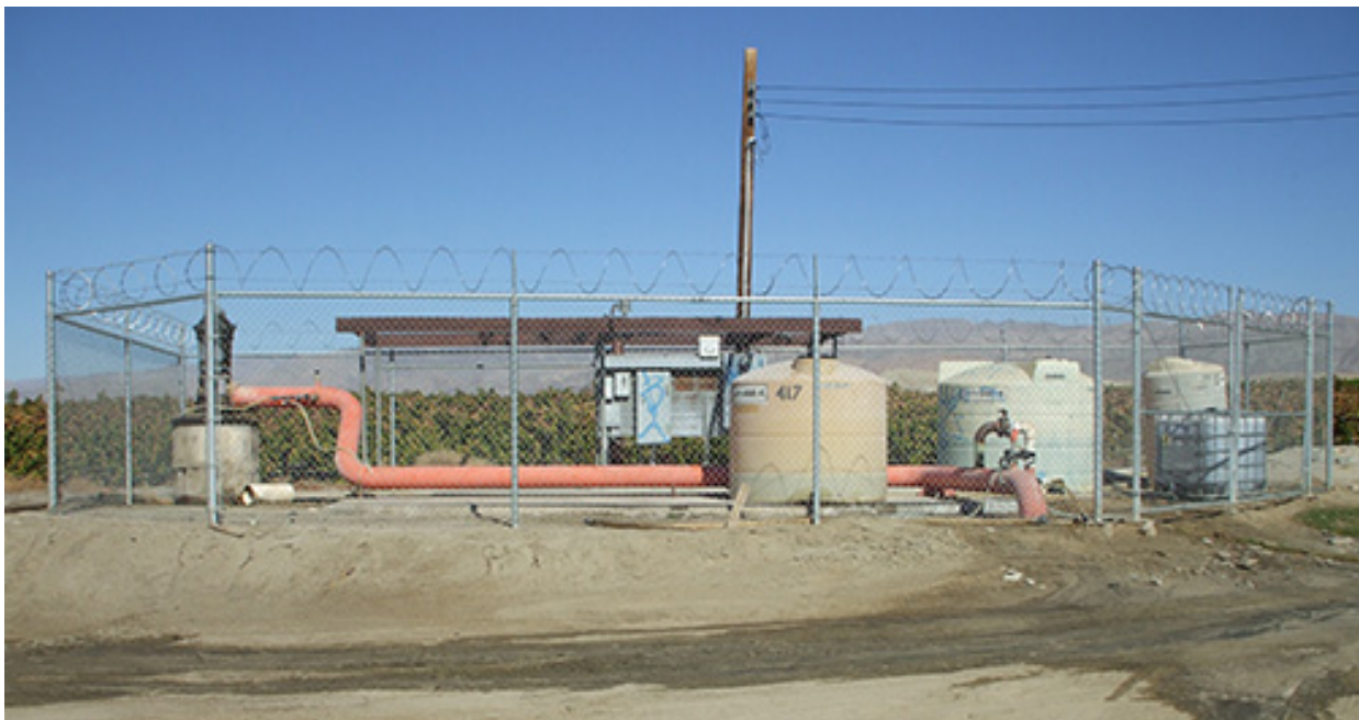
Locus C enclosed with Chain Link Fence and Barbed Wire Facing North: note old well with pump at left, linked to irrigation pipe with 3 water holding tanks at right and electrical panel in back
