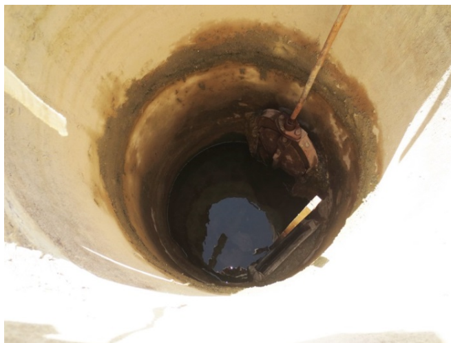
Feature 5: Probable Valve Box showing part of Valve and Valve Handle
