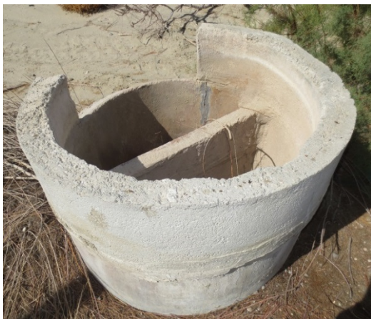
Feature 4: Constant Head Orifice
