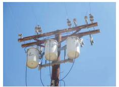
POLE MOUNTED TRANSFORMERS NEAR THE WATER RETENTION POND, TYPICAL OF THREE ON THE PROPERTY
