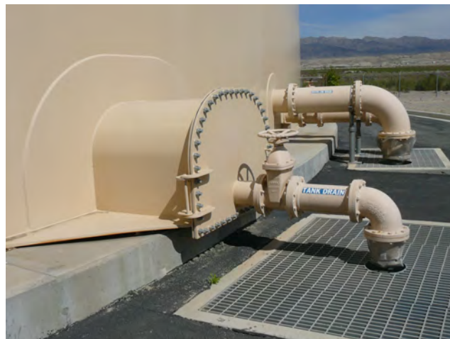
15. Shell Manway #3 with Drain
