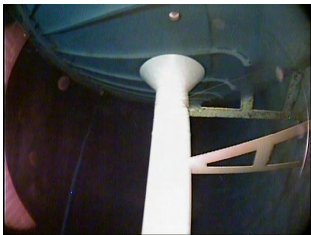
31. Interior Overflow Pipe & Bell
