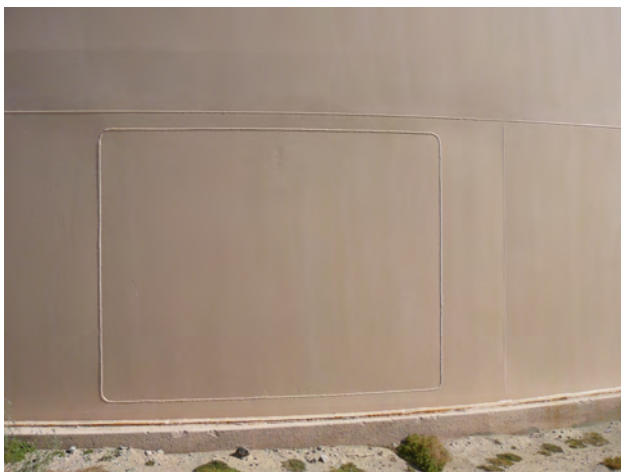
7. Exterior Shell Weld Joints
