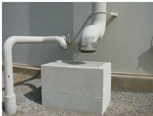
14. Overflow Drainage
