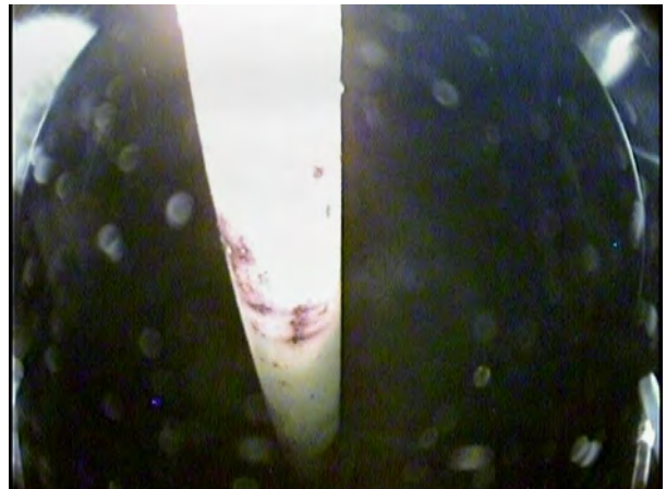
28. Center Column Corrosion
