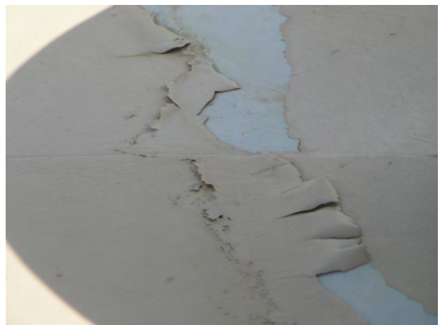
21. Paint Peeling Around Center Vent
