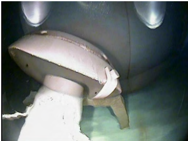
25. Interior Overflow Pipe @ Water Level
