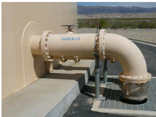
11. Overflow Pipe & Drain
