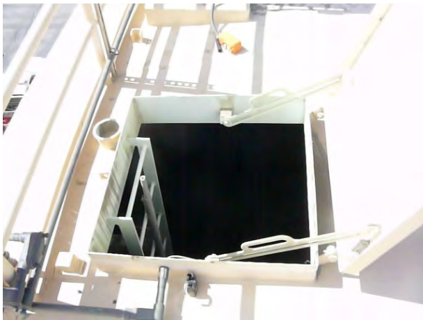
18. Roof Access Hatch
