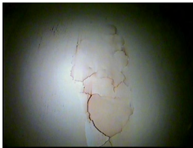
38. Wall Peeling and Flaking Coating
