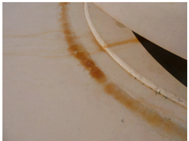
15. Paint Staining Around Center Vent
