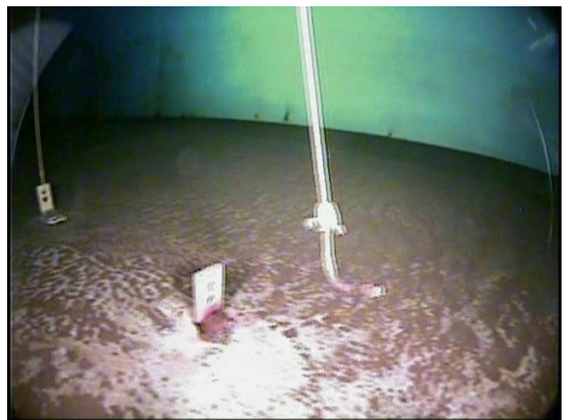
40. Float Guide Wire Detachment
