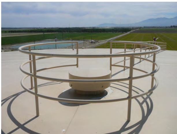
19. Roof Vent Safety Rail
