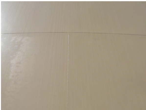
7. Exterior Shell Weld Joints
