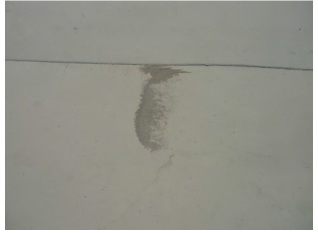
22. Roof Paddling Damage
