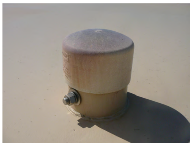
22. Roof Accessory Penetration (Typical)
