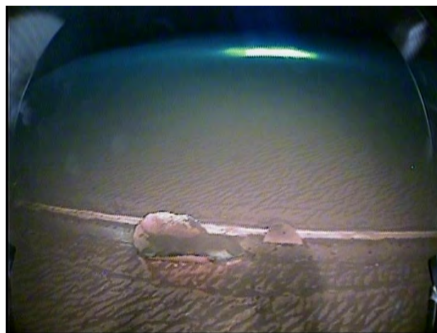
39. Floor Sediment & Debris
