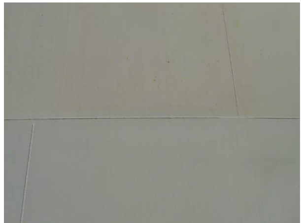
10. Shell Weld Joints
