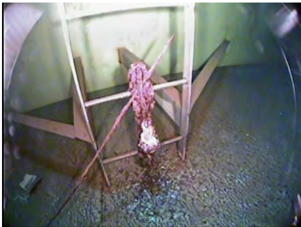
24. Failed Interior Safety Climb
