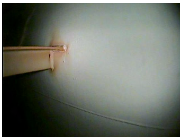
24. Interior Ladder Attachment (Run in Coating, Weld Staining)
