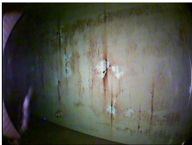
36. Wall Corrosion
