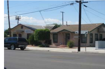
Overhead Utility Lines
