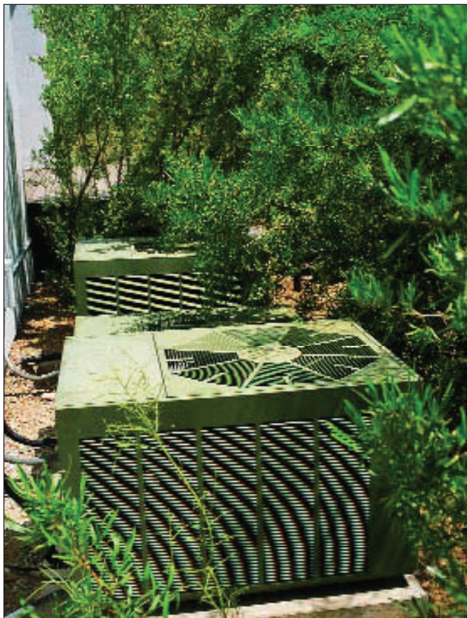
Shading air-conditioning units can reduce their workload, making them more energy-efficient.
