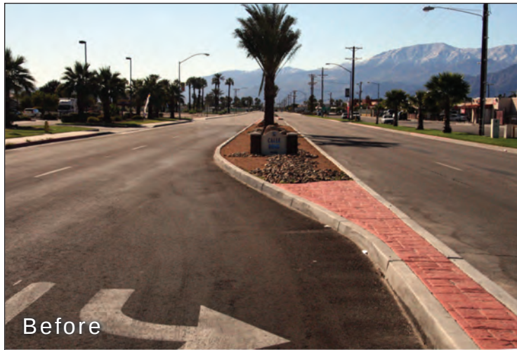
Figure 4.1: Harrison Street as it is today.
