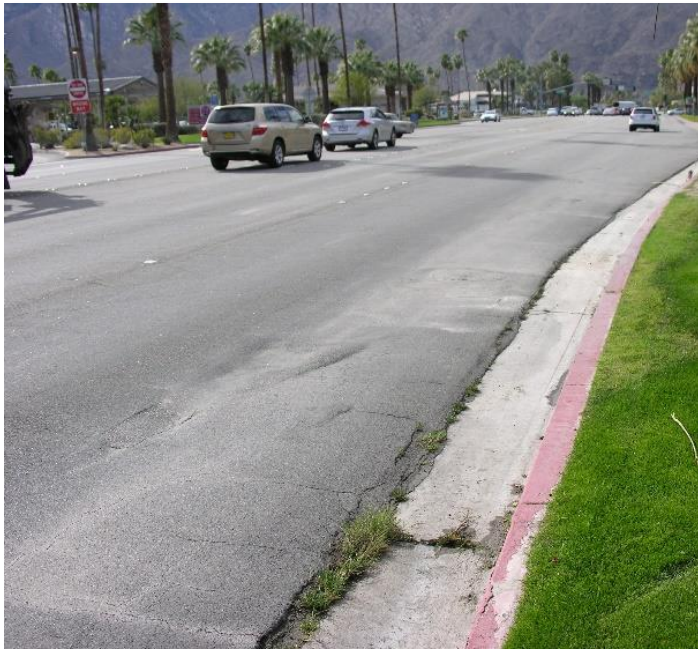
Example of Rough Pavement Section
