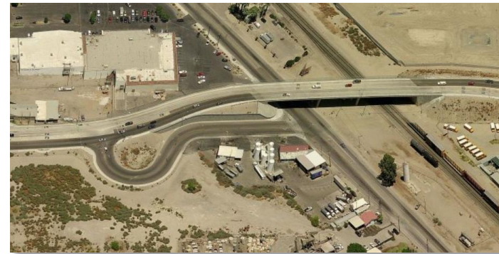
Example of New Bridge: Avenue 50 Grade Separation with State Route 111
