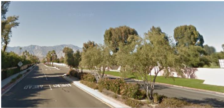
Example of Raised Median Roadway
